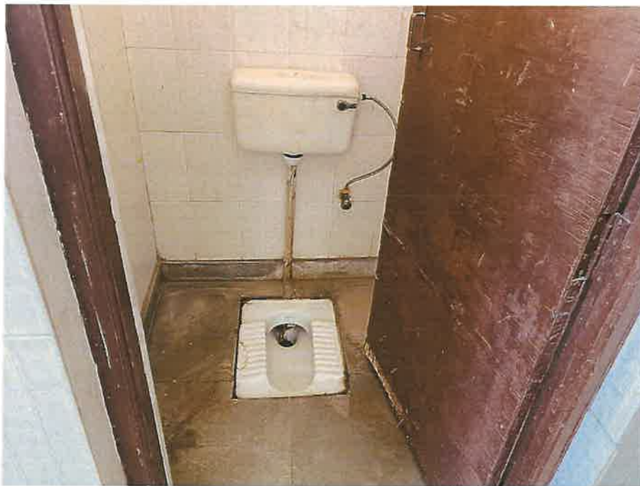
Site photograph 3 Campus Toilets
