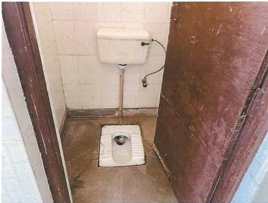
Site photograph 3 Campus Toilets
